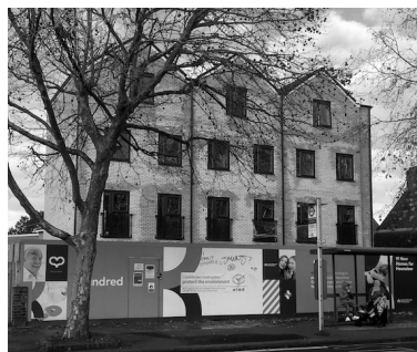
housing site on London Road is nearing completion. It includes this weirdly retro 4-storey block at the site entrance... (photo above)
